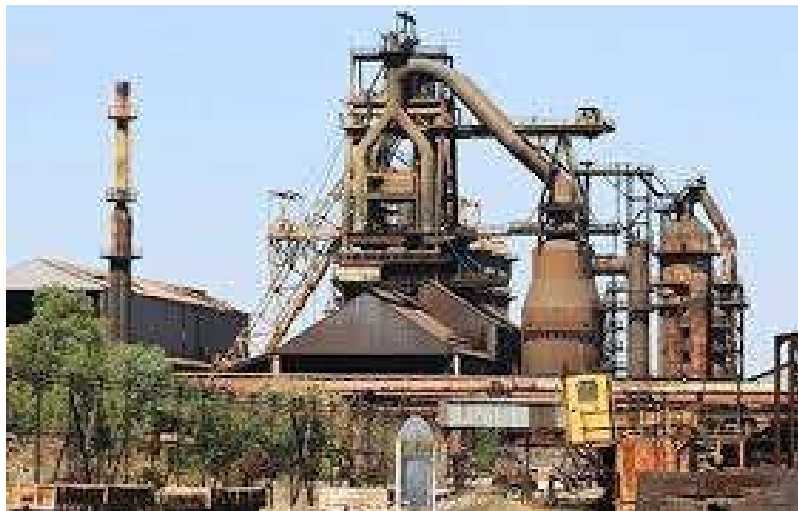
Figure 1: Ajaokuta failed steel plant
